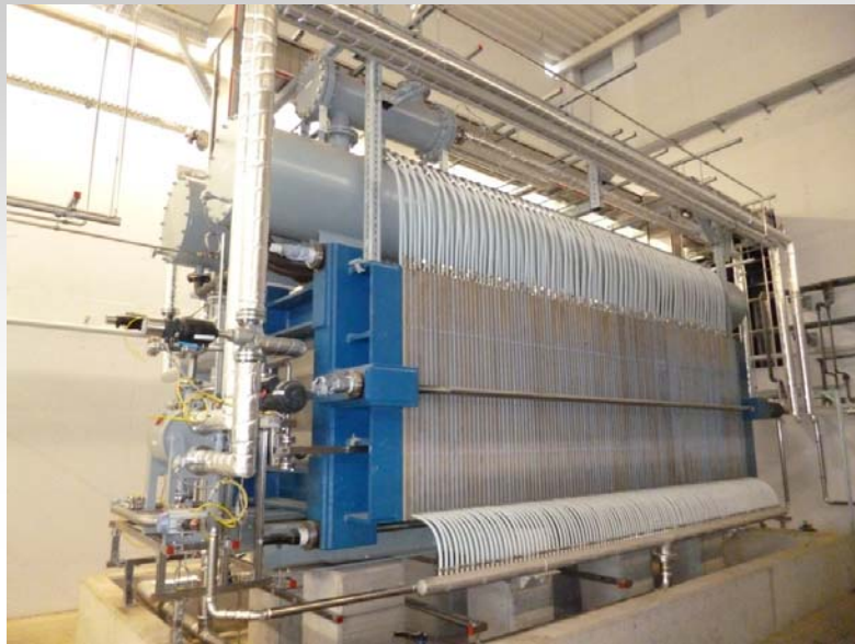
Electrolyzers (3 x 2 MW)
